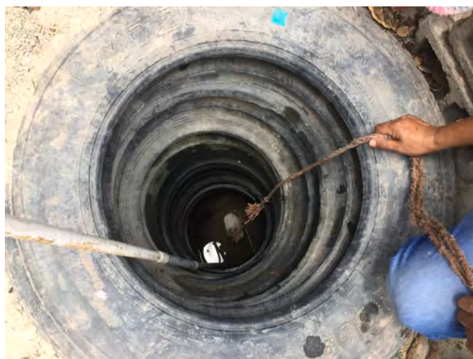
Fig. 3. Household well with tires providing structural support. The white tube on the left leads to a pump that transports water from the well to a storage container in the yard. The rope is attached to a bucket for removing water from the well. The tires above the water level in the well often contain water that provides Ae. aegypti larval habitat.
